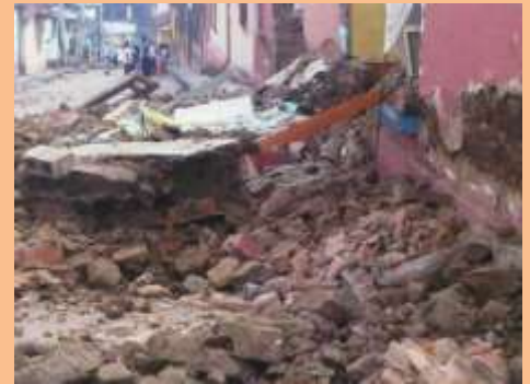
A recent earth tremor caused damage
